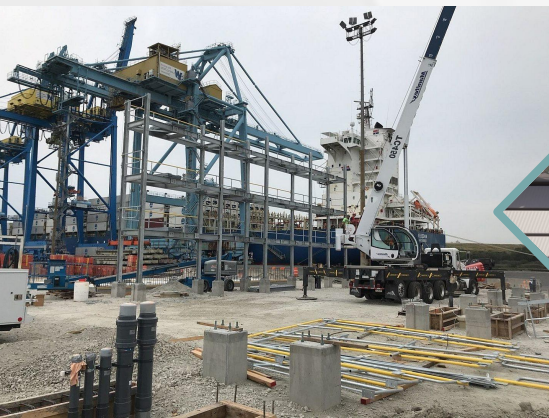
Real photo of reefer rack construction phase
